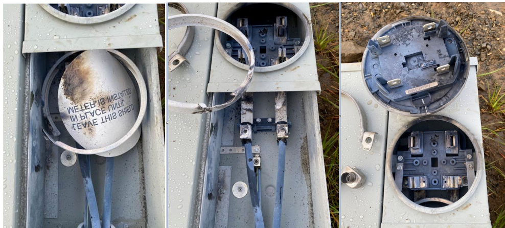
Factory provided meter ring left inside meterbase
