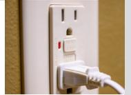
Ground Fault Circuit Interrupter (GFCI) outlets protect users from electrical shock in high-moisture areas. That's why they're required in kitchens and bathrooms, among other locations.
