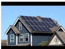
Building with Solar Panels
