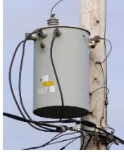
Pole mount Transformer
