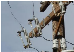
Fuse on a power pole
