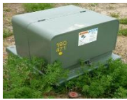
Pad mount Transformer
